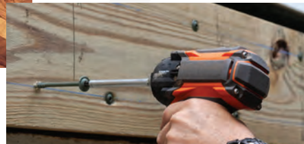
Deck Ledger Attachment
